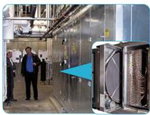
Dedicated outdoor air ventilator uses an ARI certified total-energy wheel to recover energy between the exhaust and outdoor airstreams.
