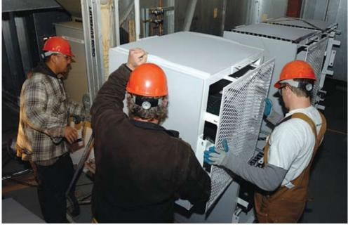
Cells are easily stacked together to form a five wide- by three-high fan array.
