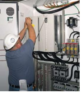
Fan speed is controlled by one variable-frequency drive with another for standby.
