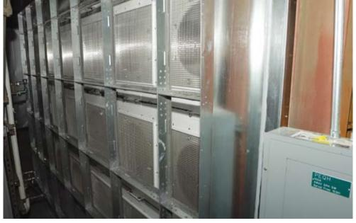
Shown is an inlet side of one five-by-three fan array with inlet screen that helps reduce pre-swirl of air entering the fan.
