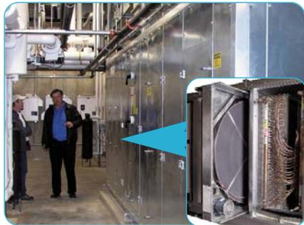
**Dedicated outdoor air ventilator uses an ARI certified total-energy wheel to recover energy between the exhaust and outdoor airstreams.**
