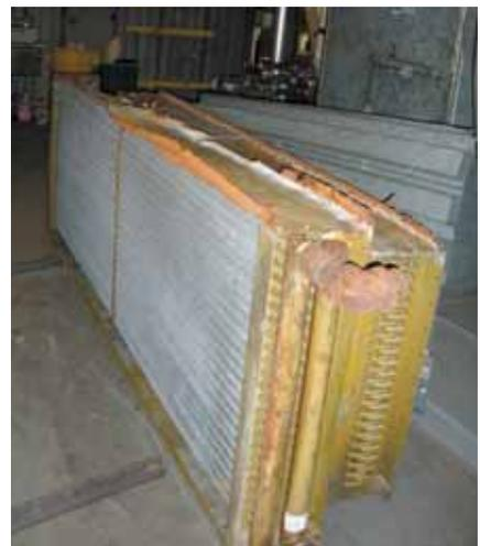
*The existing air handler was beyond its recommended service life and components had deteriorated.*
