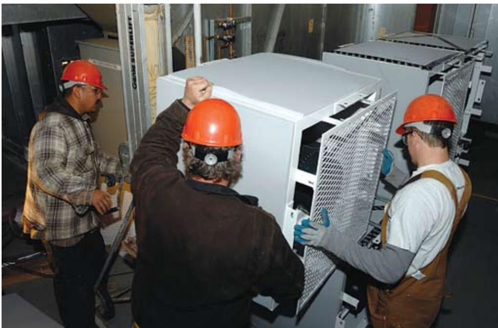
Cells are easily stacked together to form a five wide- by three-high fan array.
