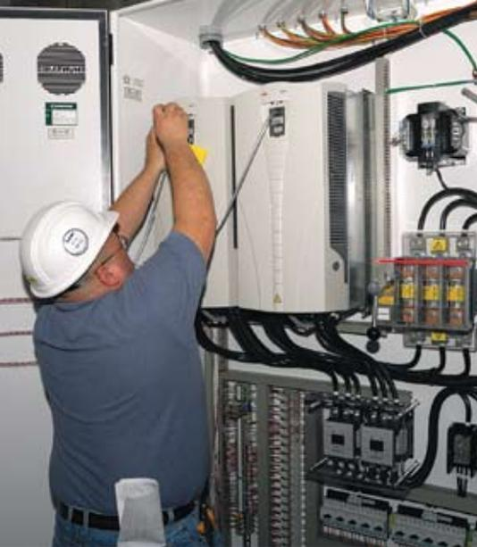
Fan speed is controlled by one variable-frequency drive with another for standby.
